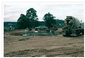
Building of the large water tank
